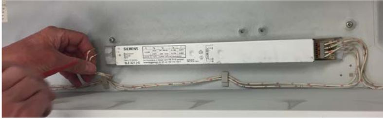
Step 1: Connect mains line "L" to fuse with one wire
