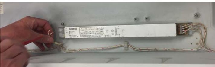
Step 1: Connect mains line "L" to fuse with one wire using a WAGO connector
