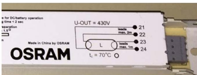
Step 2: Connect second fuse line to line „21“
